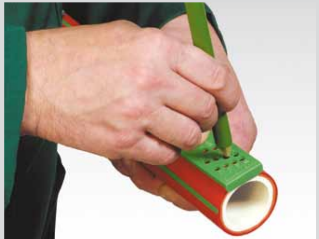
Marking of the welding depth
