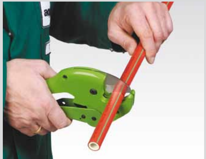
Cutting of the pipe
